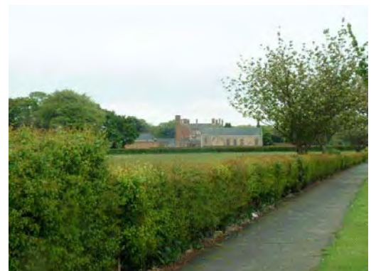
Fig. 22 View from St Mary's Walk to the rear of Acklam Hall
