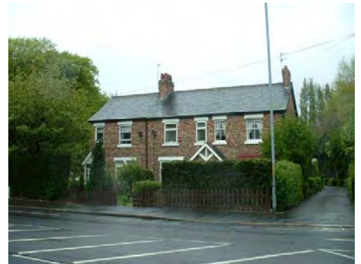
Fig.12 View of Nos. 479 - 483 Acklam Road
