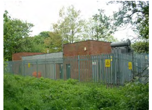
Fig.32 View of the electricity sub-station
