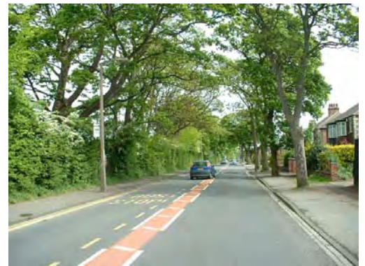
Fig. 4 View east along Hall Drive
