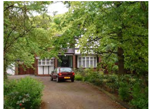
Fig. 2 View of No. 465 Acklam Road
